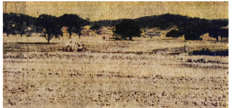
THIS VIEW taken last summer shows period when grading work was being undertaken at the area where two subdivisions were to be built. This view looking south towards Monte Maria shows graded area. The area is now dotted with houses. Novato high school is being rapidly completed nearby. Also in the immediate area two churches are being or will be built.
