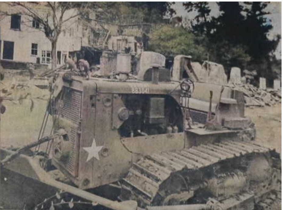
The national Guard is poised to demolish and remove the burnt out Burdell mansion at Rancho Olompali about the first of April. The Guard brought in big cats to start the demolition work at the beginning of March but rain precluded the work start. Demolition will demand much care as the old adobe inside the mansion is to be preserved as a state historical landmark.
